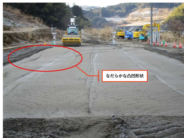
Fig. 19 2層目の出来形(凸凹形状) Second Layer Finished Shape (Rough Shape)
