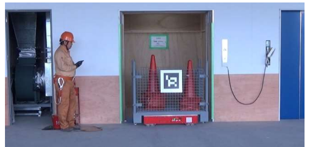
Photo 8 実験状況 Experiment in Construction Site of Shopping Center
