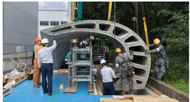
Photo 10 建方状況 Erection and Installation of Pieces
