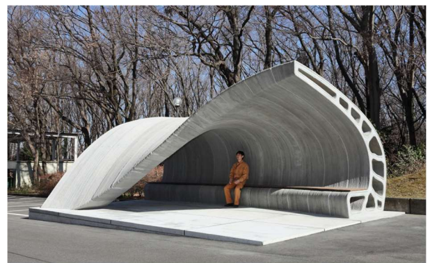
Photo 11 完成状況 Completion of Shell-shaped Bench
