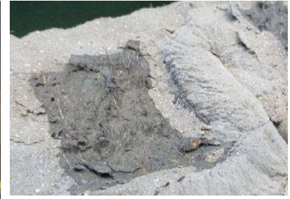
Photo 5 破壊面の拡大 (No.1) Detail of Fracture Surface (No.1)
