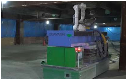
Photo 9 自律移動, 位置合わせ状況 Autonomous Movement and Alignment of Robot
