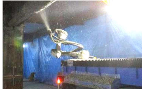
Photo 10 耐火被覆の吹付け状況 Fireproof Coating Spraying by Robot
