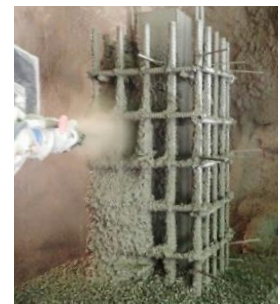
Photo 3 吹付状況(柱) Spraying (Column)
