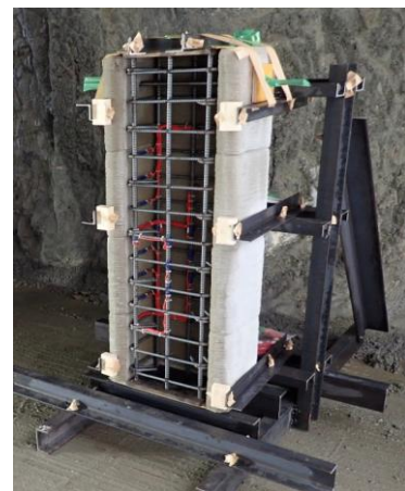
Photo 8 外殻と鉄筋配置 Outer Shell and Rebar
