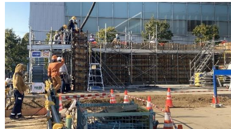
Photo 3 壁部材への打込み状況 Status of Concrete Placement on Wall Members
