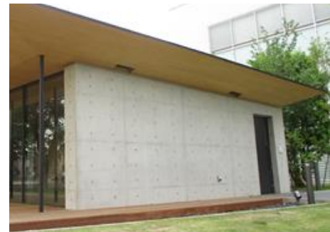
Photo 4 建物の外観 Exterior of the Building
