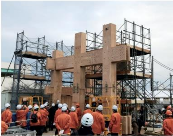
Photo 2 実大施工試験状況 Situation of Full-Scale Construction Test
