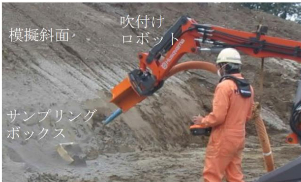
Photo 2 吹付け状況 In-Suit Test of Shotcrete
