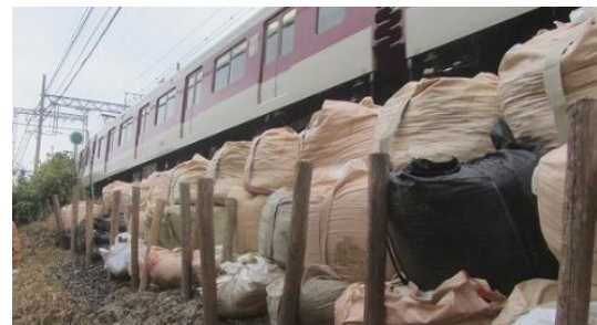
Photo 3 鉄道盛土被災後の応急復旧状況 Emergency Recovery After Disaster of Railway Embankment
