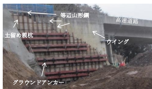
Photo 7 最終掘削完了 Completion of Final Excavation
