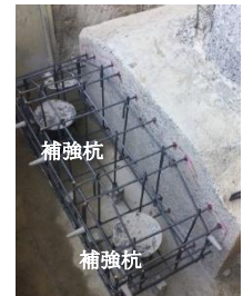
Photo 2 補強杭の 施工完了状況 Completion with Construction of Reinforcement Pile
