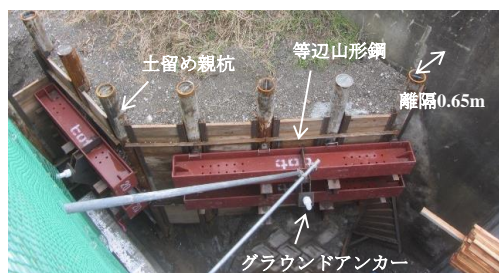
Photo 9 土留め親杭の施工完了状況 Completion with Construction of Soldier Piles
