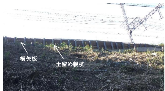
Photo 5 土留め親杭の施工完了状況 Completion with Construction of Soldier Piles
