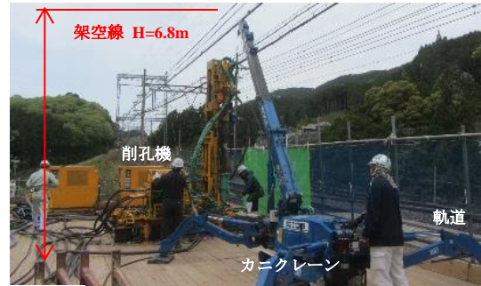
Photo 4 鉄道営業線での二重管削孔状況 Double Tube Excavation Nearby Railway
