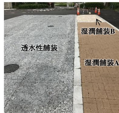
Photo 1 試験施工範囲 Test Construction Area
