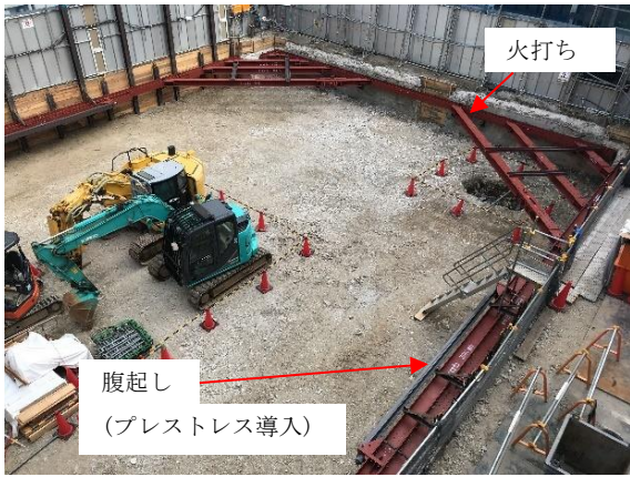
Photo 1 鋼製支保工の架設状況 Installation of Steel Support Works
