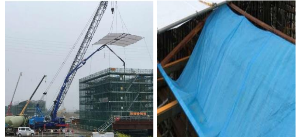
Photo 1 シートによる降雨対策の例 Example of Covering Concrete with Sheets to Prevent Damage from Rainfall
