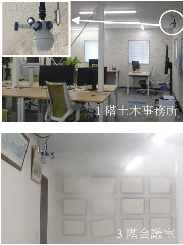
Photo 1 適用状況 Application Status
