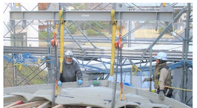
Fig. 20 3DP製デッキの建方 3DP Deck Laying on the Roof Slab
