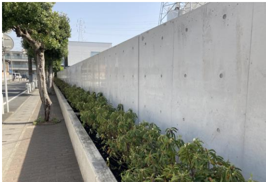
Photo 4 RC外壁の外観 Exterior of the RC Wall
