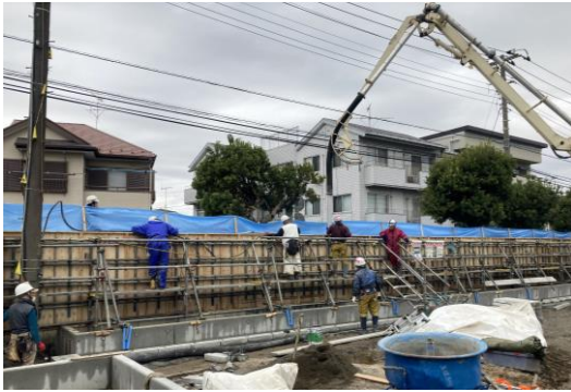
Photo 3 打込み状況 Status of Concrete Placement
