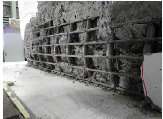
Photo 2 補強軸方向鉄筋の座屈 (4-3試験体) Buckling of Additional Rebar (No.4-3)
