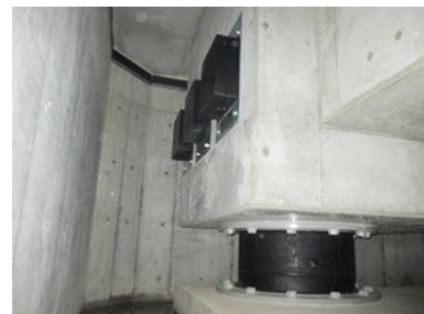
Photo 2 免震フェンダーを設置した建物 A Building Where Menshin Fenders were Actually Installed
