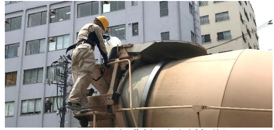
Photo 4 硬化促進剤のあと添加状況 Addition Status of Hardening Accelerator
