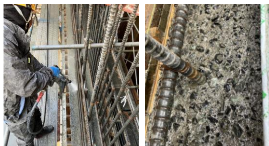
Photo 6 洗出し状況と洗出し後の打継目 Situation of Aggregates Expose and Joint Surface after Aggregates Expose
