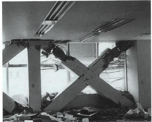
Photo 1 SRCブレース被害状況(6階) Damage of SRC Brace (6th Story)
