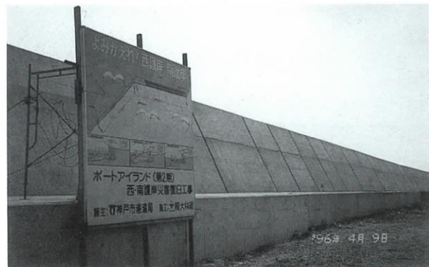
Photo 2 復旧状況 (P.I. II 西・南護岸) Restoration Work (No. 1)
