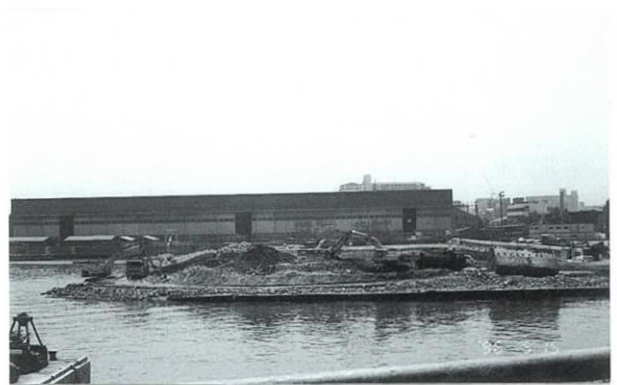
Photo 7 復旧状況 (神戸商船大学) Restoration Work (No. 4)
