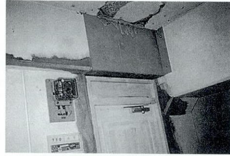
Photo 10-2 鉄板の設置 Installing the Steel Plate
