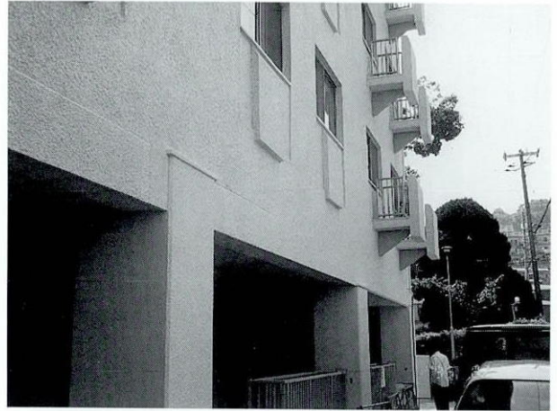
Photo 4 補修・補強工事完了 Completion of Repair and Strengthening Work
