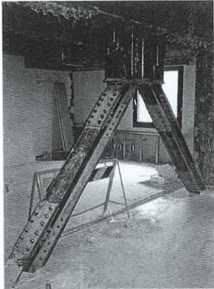
Photo 7 Y形ブレース取付 Attaching Y-Shape Brace
