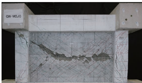
鉄筋モルタル造耐震補強壁の最終破壊状況 The Ultimate Failure State of Reinforced Mortar Retrofit Seismic
